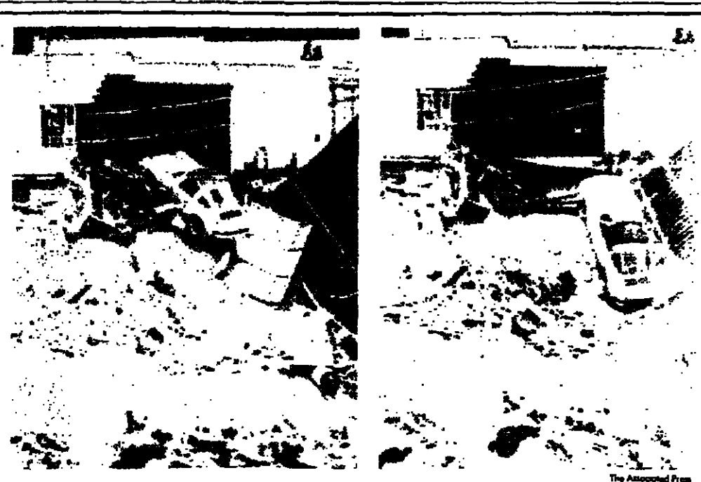
A car falls out of the back of a crumbling building into a large, growing sinkhole in Florida.
